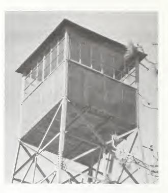
Figure 147. The cab on the Coronado's West Peak lookout (Aermotor MC-40).
